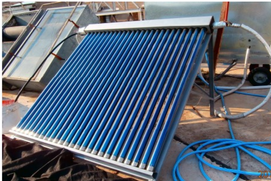
Figura 1. Colector de tubos evacuados “water in glass”
